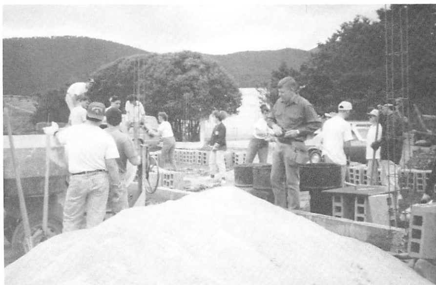
Corey Bontrager uses a level to be sure the blocks are properly aligned while Shanna Moyle fills the joints with cement.
